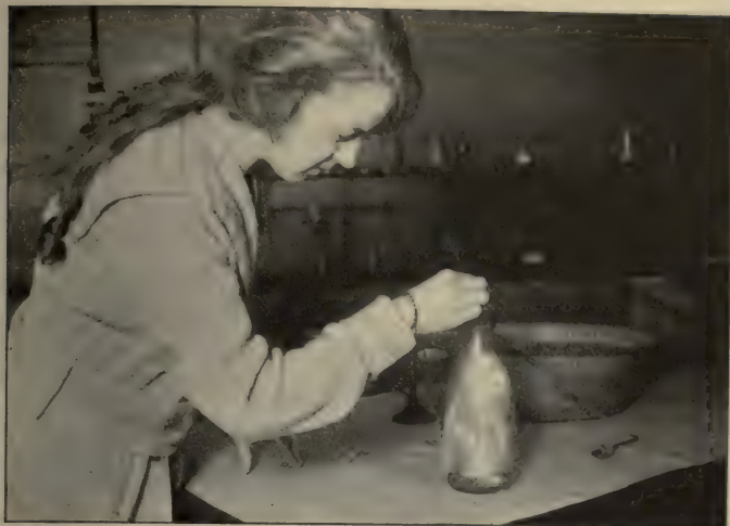
FIG. 166. The iron really burns in the jar of oxygen.
